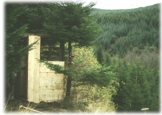
doe box under construction
